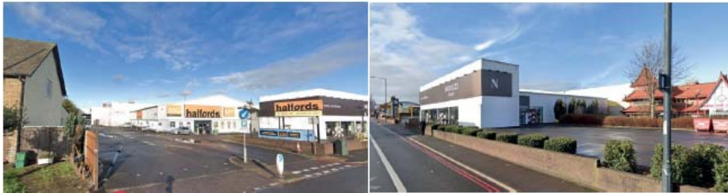
Fig 3 – Photos of site
